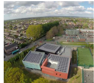
6. The Fuse, Partington (49.82 kWp)
