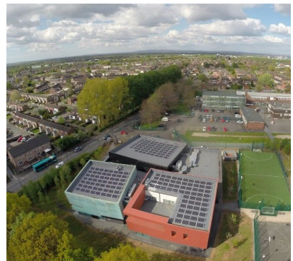
6. The Fuse, Partington (49.82 kWp)
